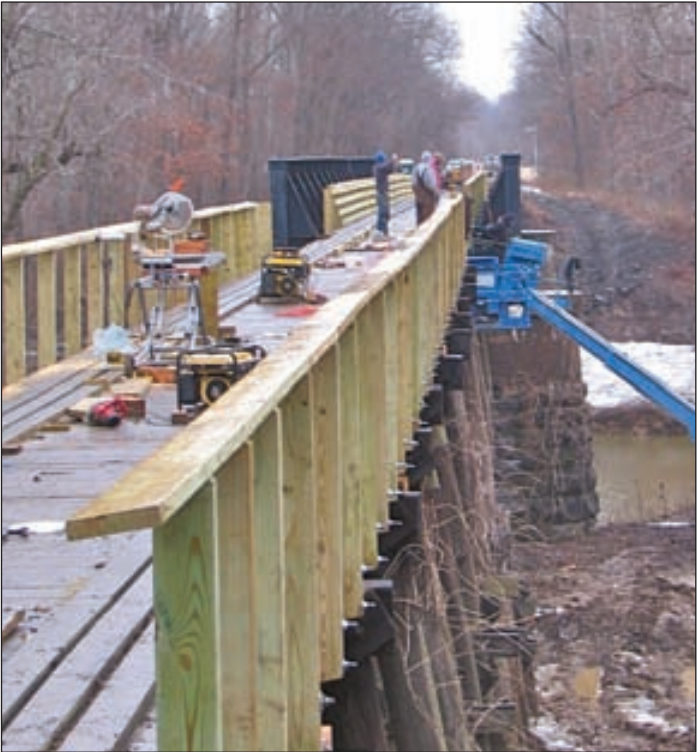
PHOTO BY DARYL K. Tabor, THE PRESS Workers put the finishing touches earlier this month on the new decking of the Blackford Veterans Memorial Bridge spanning the Tradewater River that divides Crittenden and Webster counties. The bridge, originally built for a railroad in 1887, is part of the Blackford Walking Trail.
